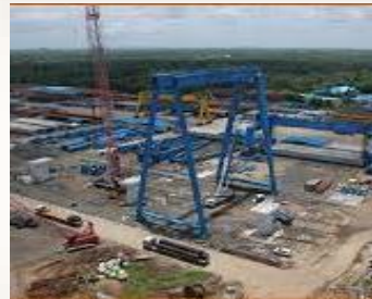
Casting Yard Mira Road, Mumbai
