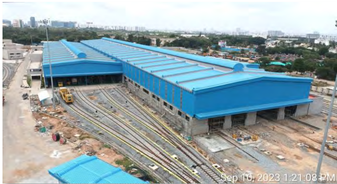
BMRCL (METRO SHED) - BANGALORE
