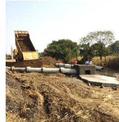
Village infra development
