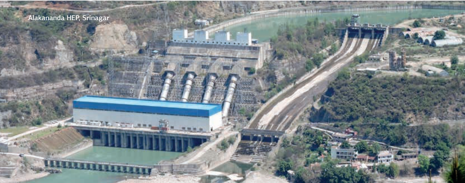
GVK Power (Goindwal Sahib), Punjab
