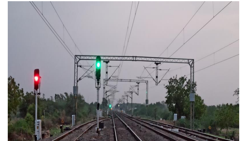
Automatic Block Signaling
