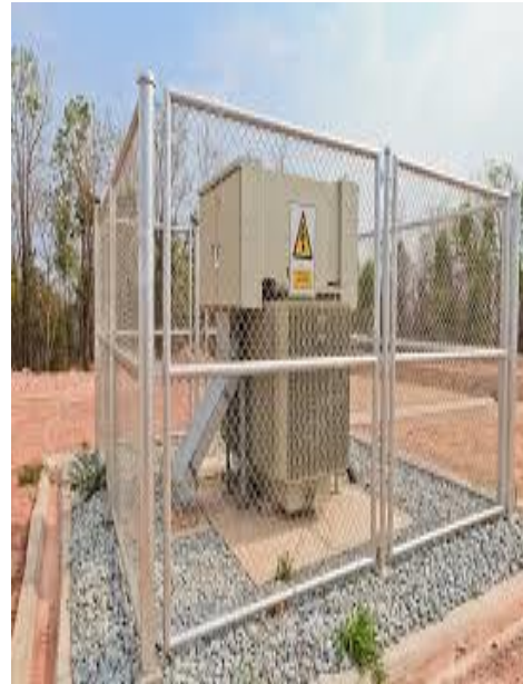
Fencing/ Protective Screen
