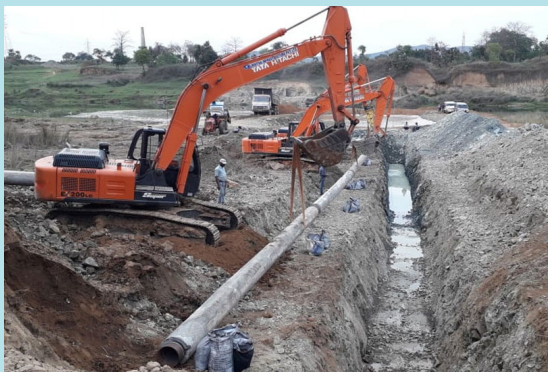
Cross-Country Pipeline Projects (CCP)
