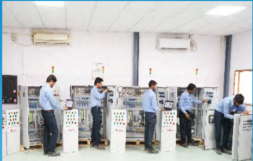
Industrial Automation: Control Panel Building
