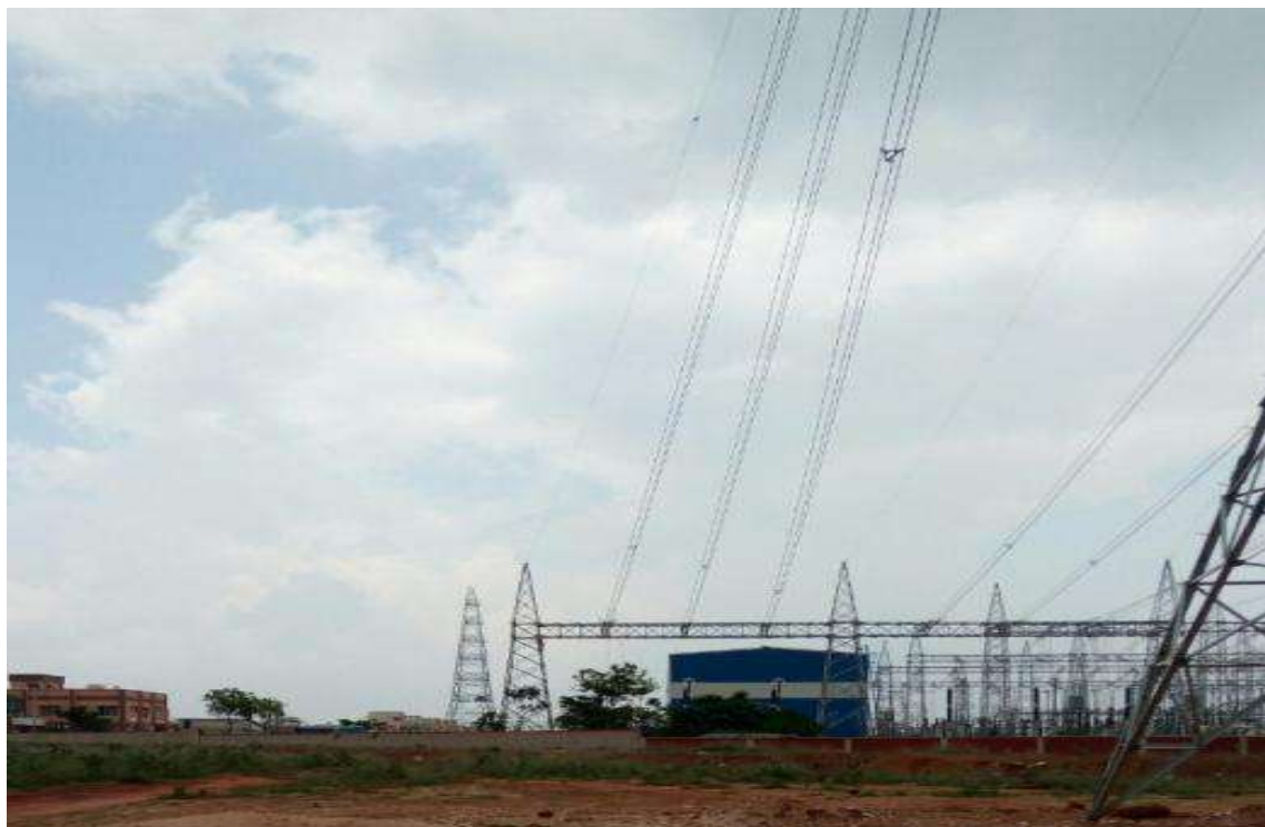
Sundergarh PGCIL substation – Gantry connection complete
