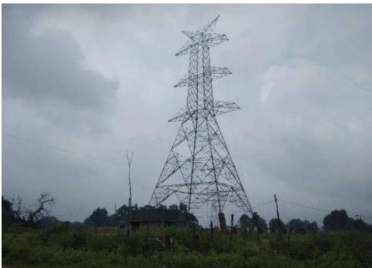
108/4 to 108A/0 – Tower erection complete
