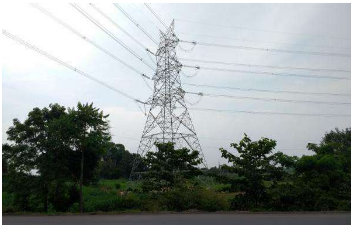
Location 32/0 – Road crossing, Erection and stringing complete
