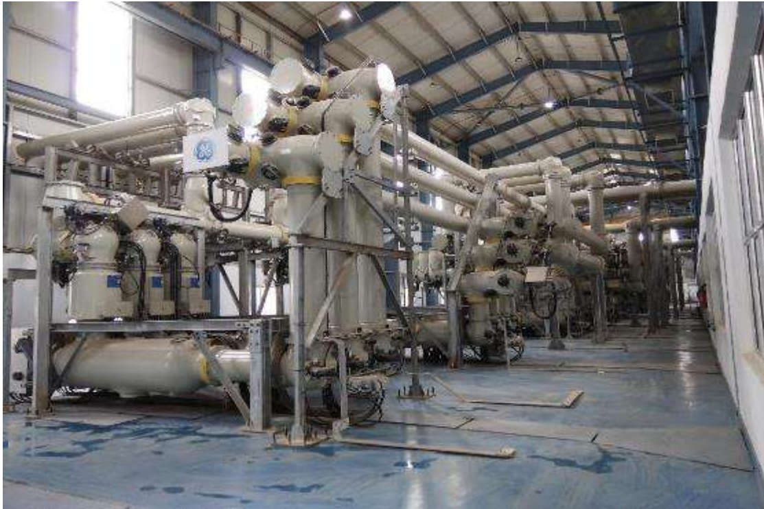
400 kV GIS sub – station, Equipment installation complete, tested and charged
