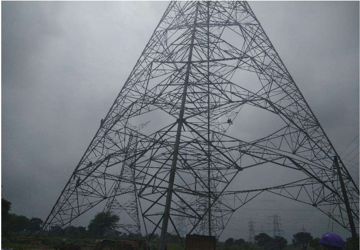
Location 104A/0 – Tower erection in progress
