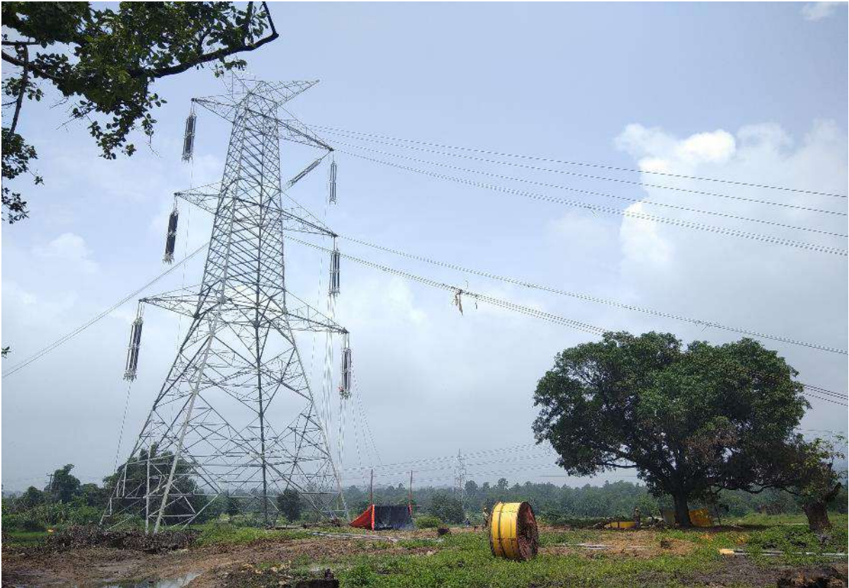
Location 115/0 – Stringing works are in progress
