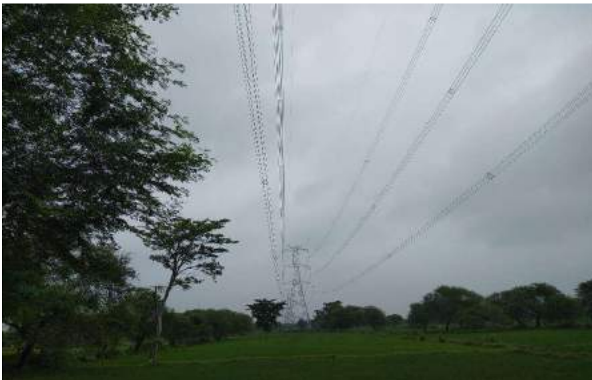
Stretch 1/0 to 4/0 – Stringing complete
