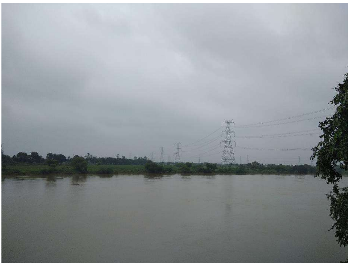
Section 2/3 & 3/0 – river crossing stringing complete
