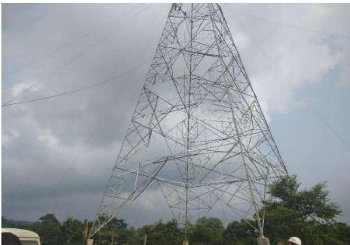
Location 108/3 – Tower erection in progress
