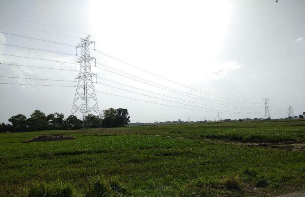
Stretch 20/3 to 30/9 – Stringing complete
