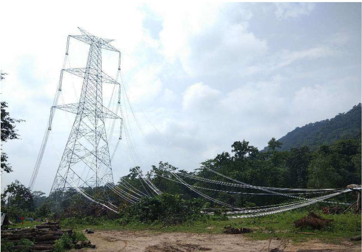
Stretch 115/6 to 116A/0 – Stringing in progress
