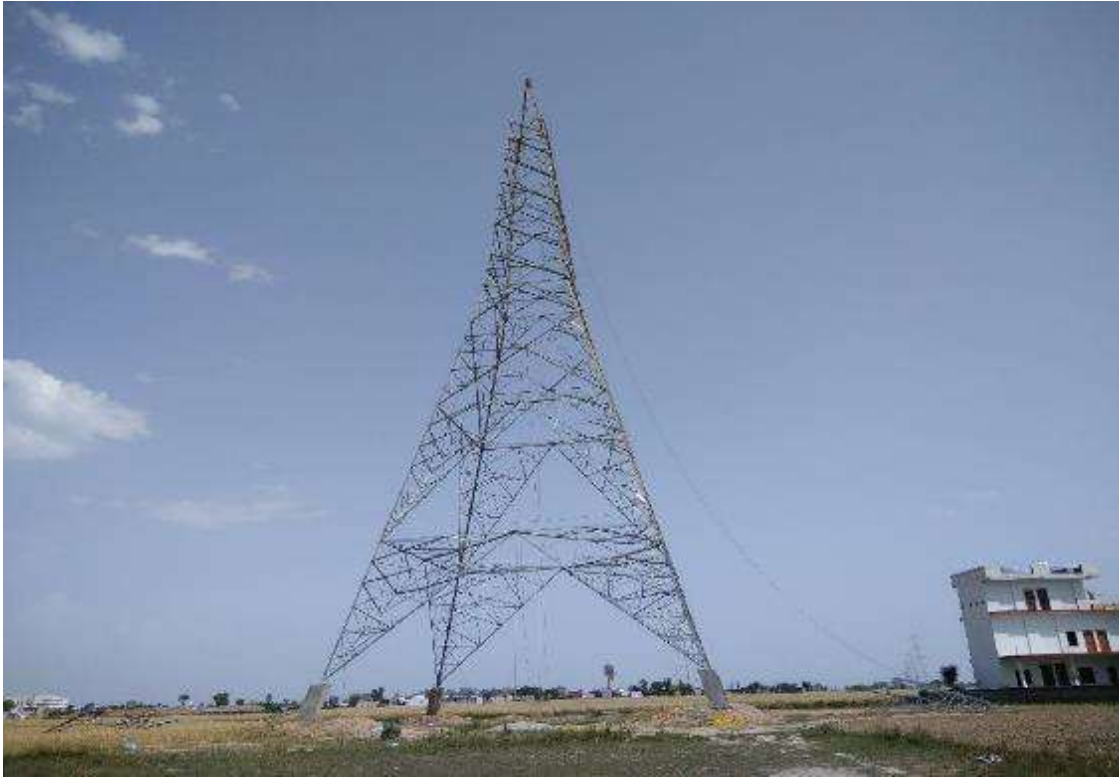
Location 34/0 – Tower erection in progress
