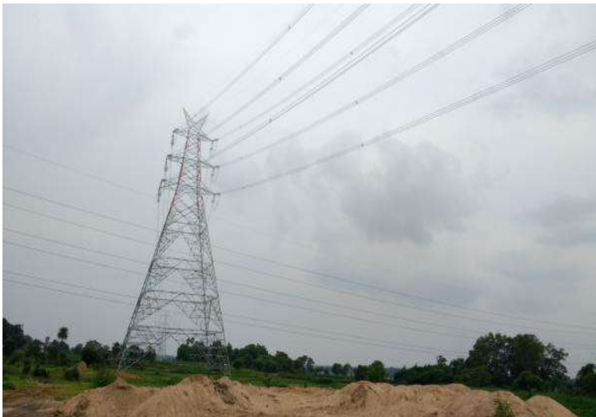
Stretch 32/0 to 33/0 – Stringing complete
