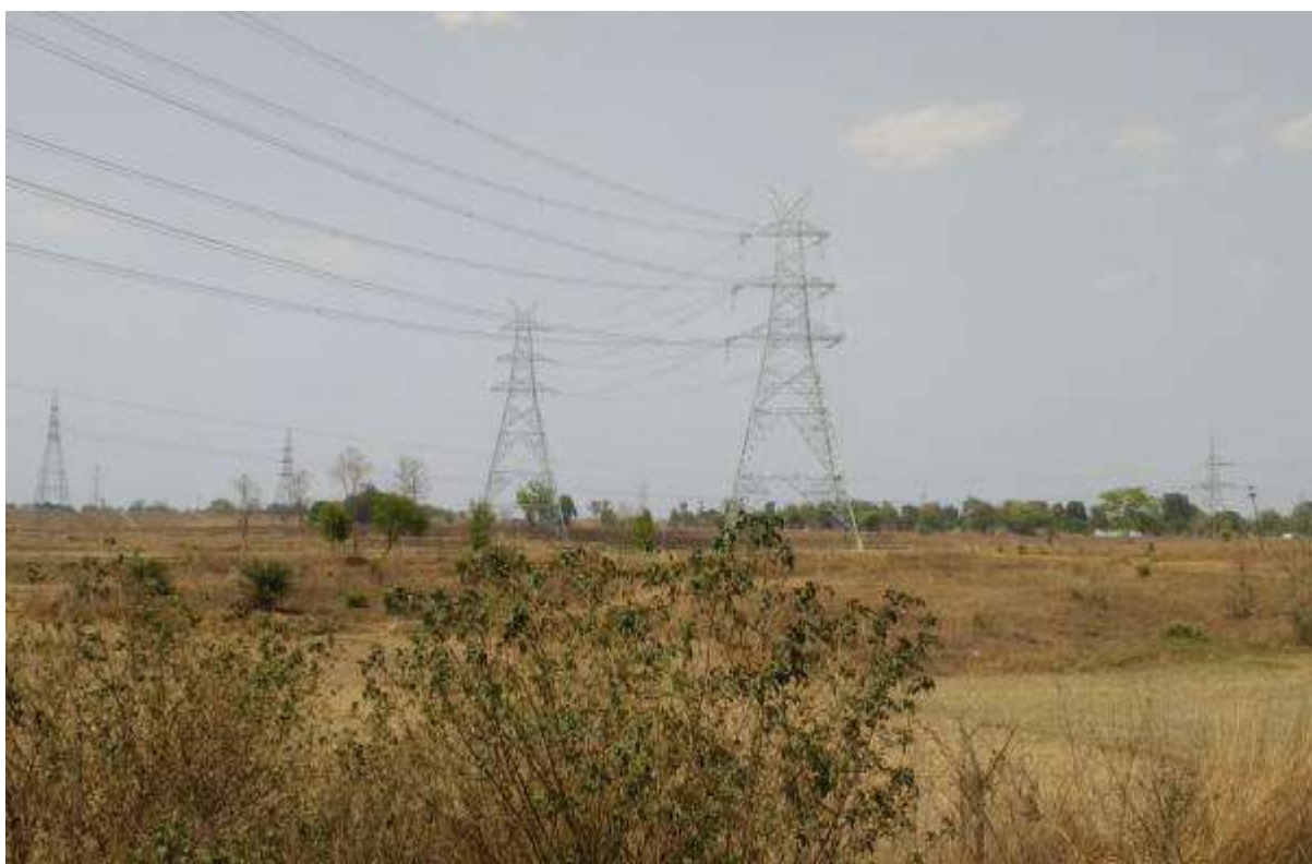
Stretch 30/0(DD+18) to 35/0 (DC+0) – stringing complete
