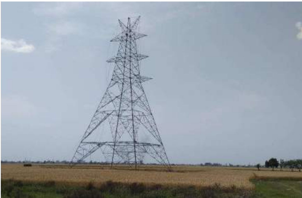
Location 35/0 – Tower erection progress
