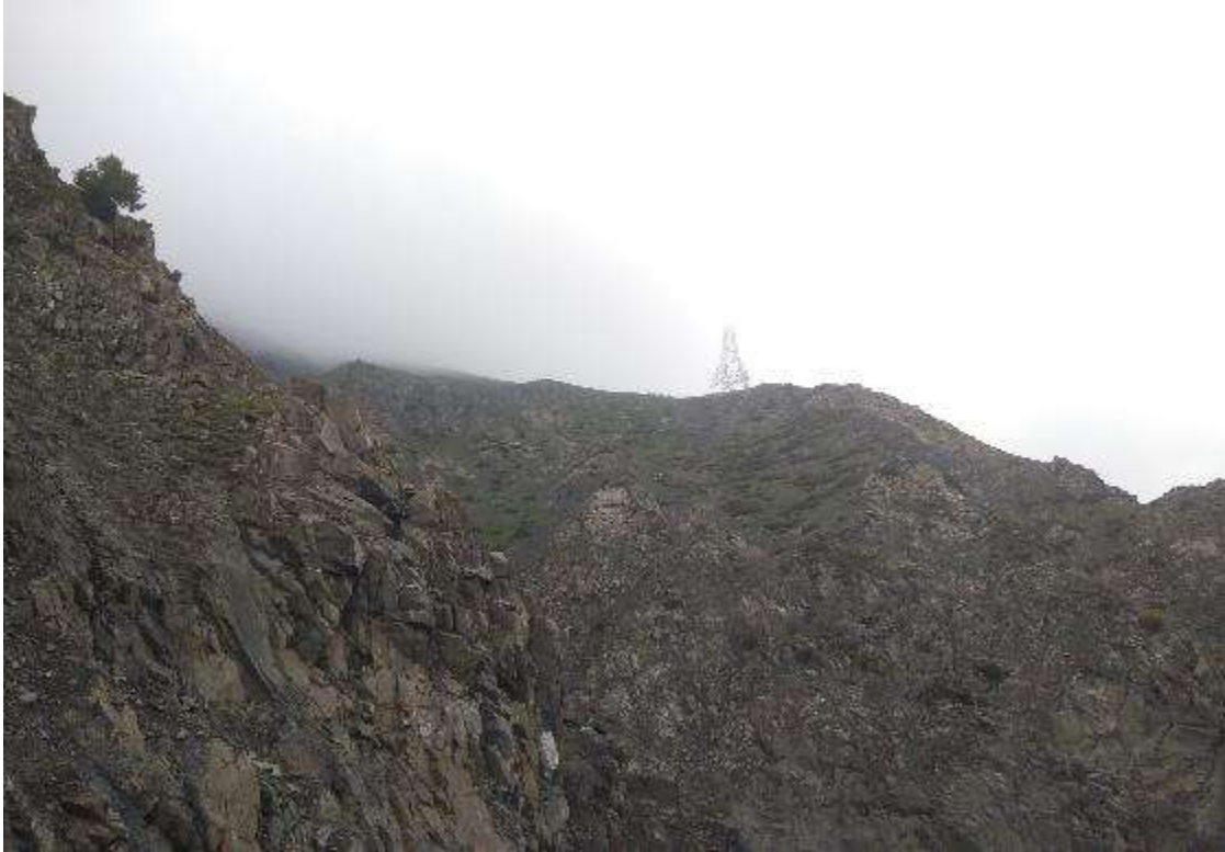
Location 338/1 – Tower Erection in progress
