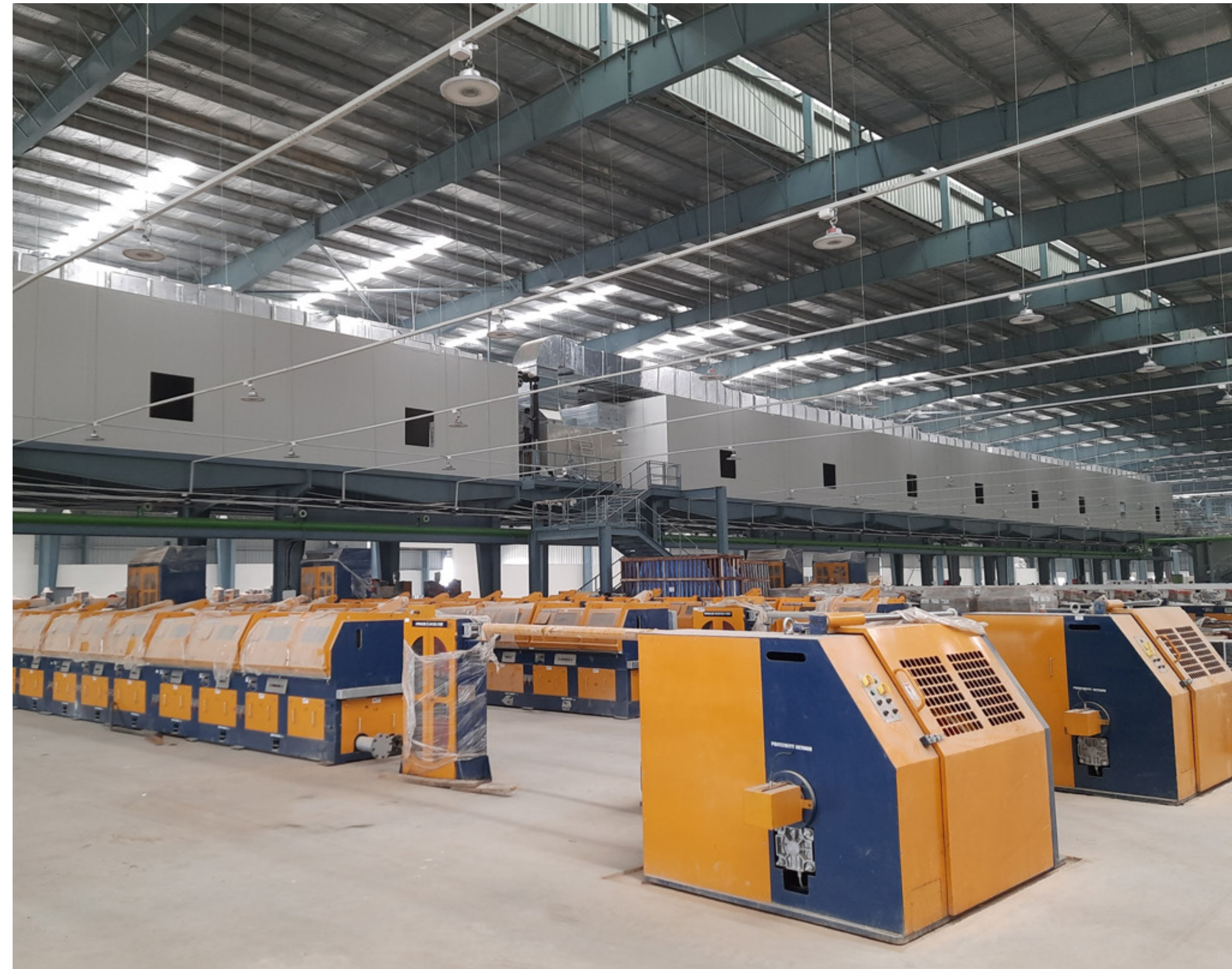
▲ Chennai plant commissioning underway
