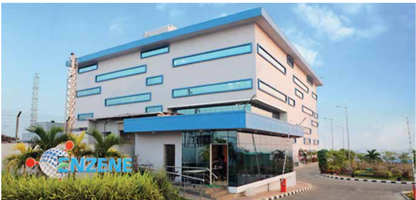
Manufacturing facility of Enzene Biosciences at Pune, India
