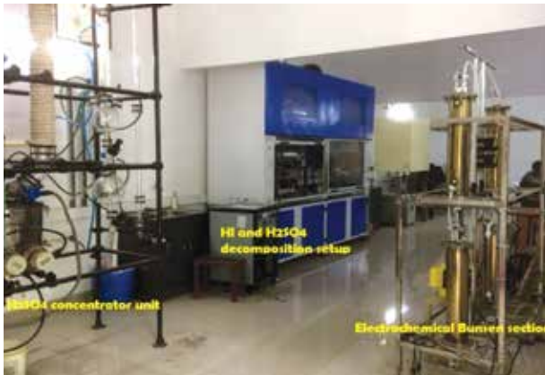
I-S closed loop cycle facility
