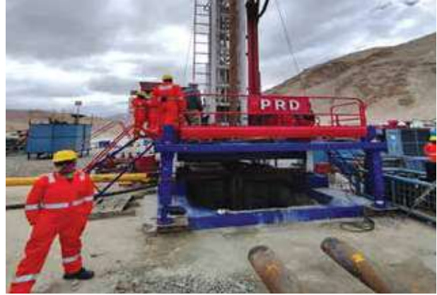
Geothermal drilling site at Puga, Ladakh
