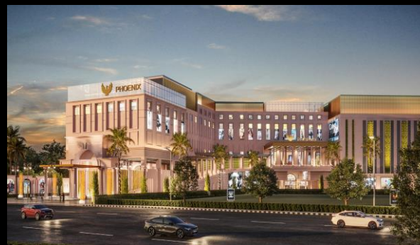
Under-development mall at Kolkata
