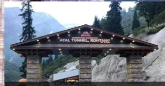
Atal Tunnel, India
