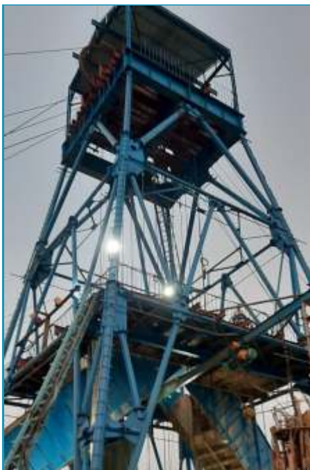
Vertical Shaft at MOIL's Mine
