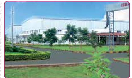
NANDIGAON - Near Hyderabad, Telangana Product line: 2V/12V - PLT and Tubular flooded batteries
