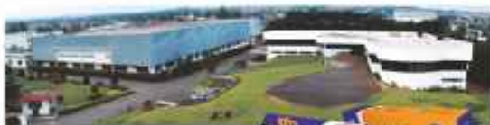
Menon Bearings plant at Kolhapur,
