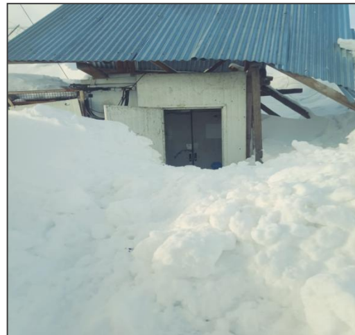
Picture showing site restoration activity in JK
