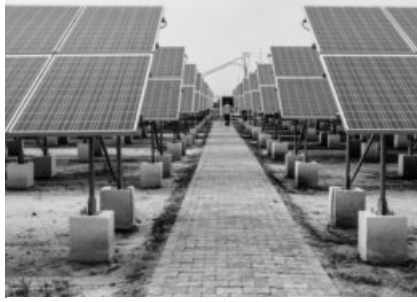
UP is planning to install rooftop solar plants and solar parks to achieve the target
