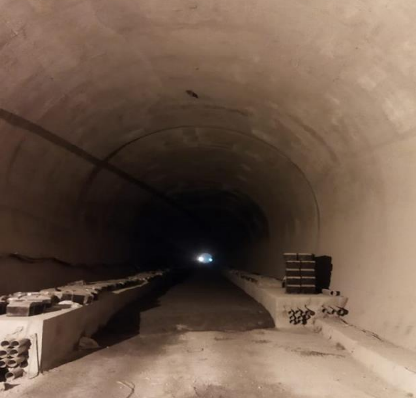
Main Tunnel 2 nd stage concrete
