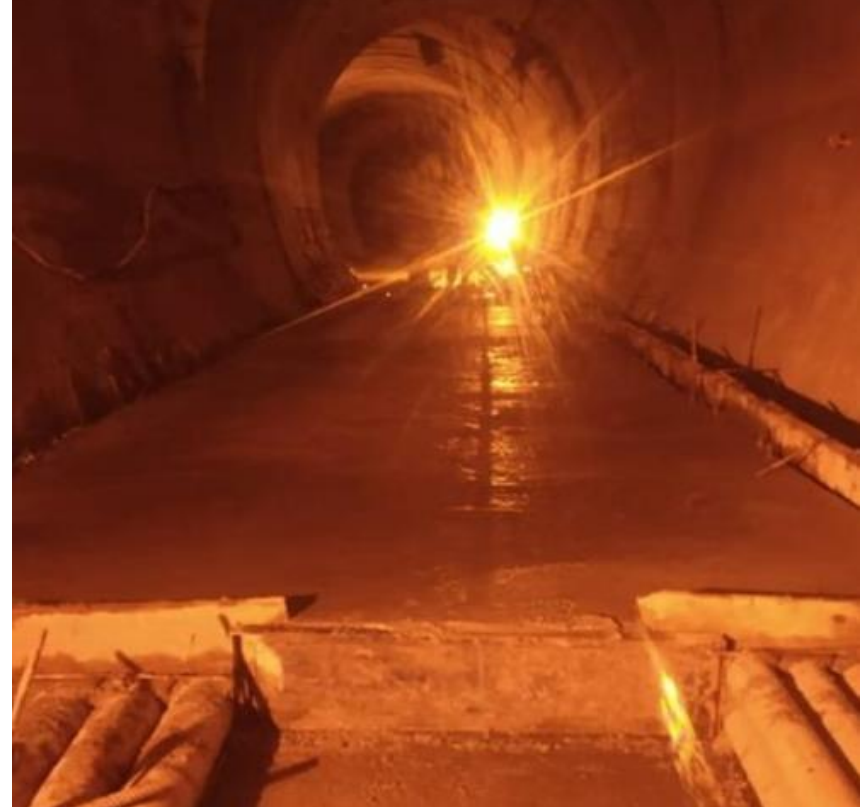
Escape Tunnel 2 nd stage concrete
