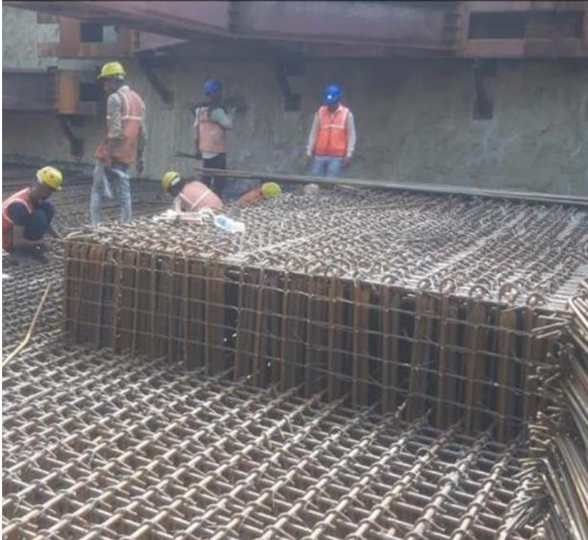
Station Concourse Slab
