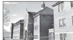
A 1970 image of the school in British Columbia, Canada
