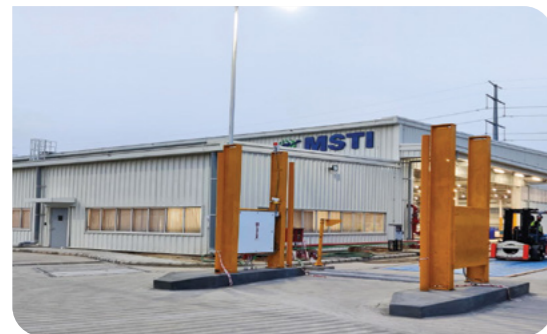
A view of MSTI facility
