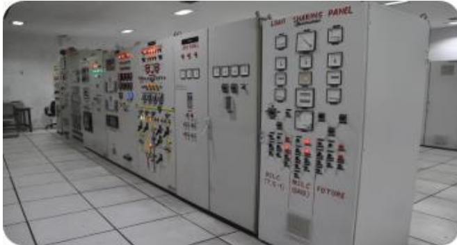
Cogeneration Control Panel
