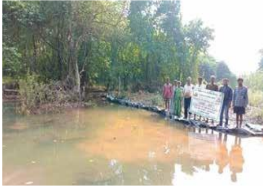
Check Dam: Moravane, Chiplun, Ratnagiri
