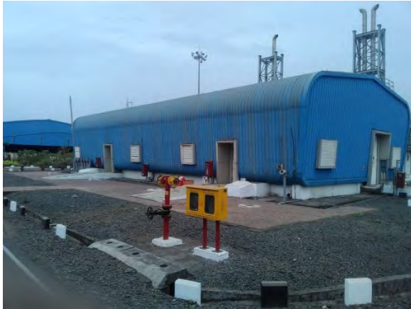
CS - 8 Electric Sub Station
