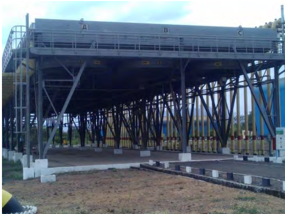
CS - 8 Gas After Cooler
