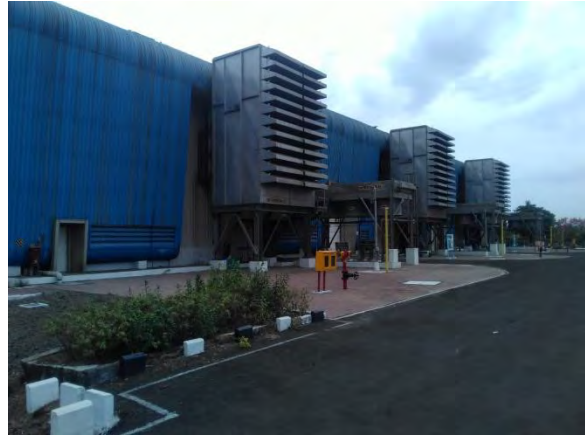
CS - 8 Compressor House
