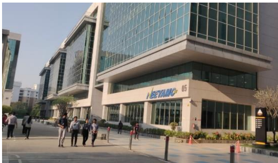
External view of the buildings at subject property
