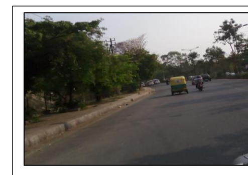
View of the primary access road
