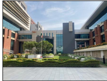
External view of the SP
