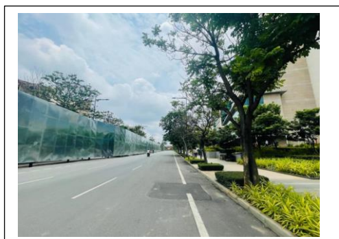
View of internal access road
