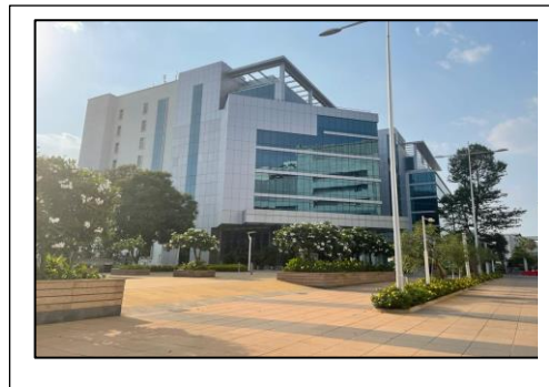
External view of the SP
