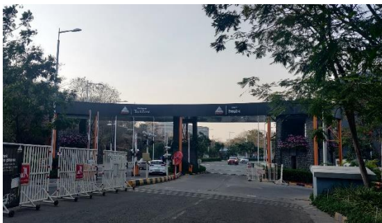
View of entry gate to subject property
