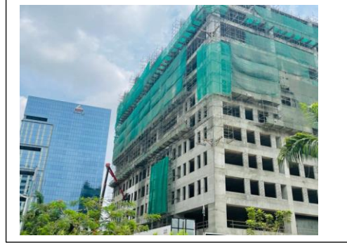
External view of Block M3 at the SP
