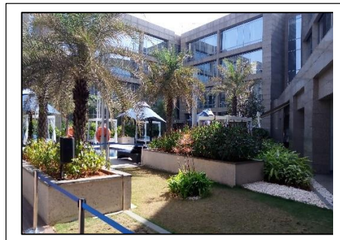
External view of the SP
