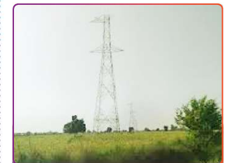
765kV Ghatampur TPS-Agra SC line
