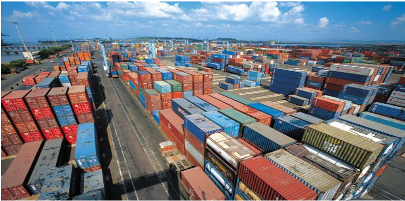
Nhava Sheva International Container Terminal (NSCIT)
