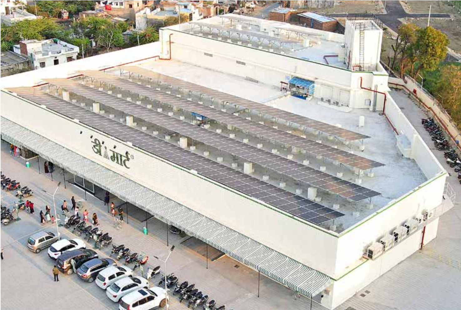
Rooftop Solar Panels
