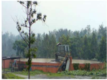
Primary Clarifier - Pulp
