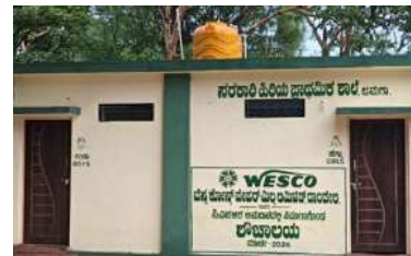
Toilet Blocks - Govt. Hr. Pr. School, Jamga Village
