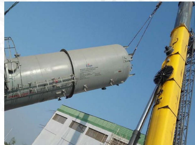
Fabrication & Erection of Equipments
