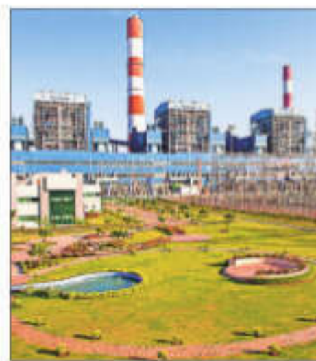
Adani Power exports electricity to Bangladesh from its coal-fired Godda plant in Jharkhand
