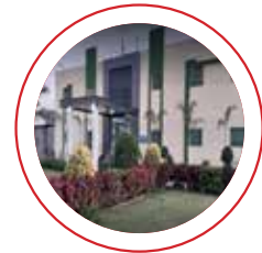
Parbhani Plant Capacity : 190 MT/ Day
