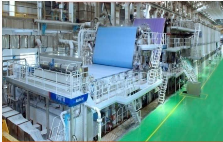
FINISHED PAPER – 1,82,400 TPA
