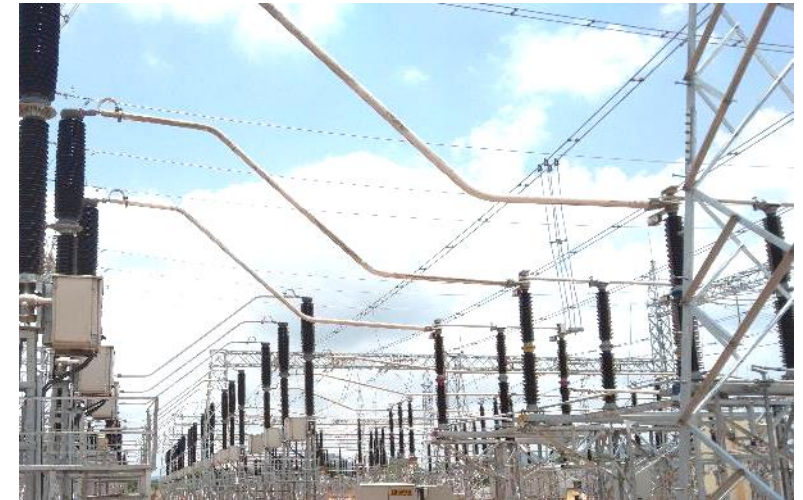
MP Power Transmission Package-II: Design, Engineering, Procurement, Supply, Construction, Installation, Testing & Commissioning for 04 nos. 220kV, 132kV & 33kV Substations
