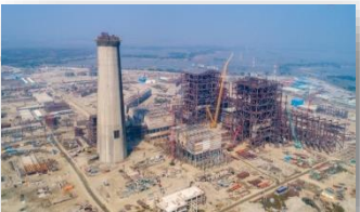
2X660 MW at Rampal, Maitree, Bangladesh-BIFPCL
