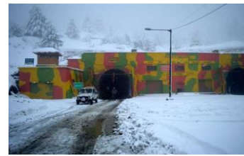
Jawahar Tunnel, J&K
