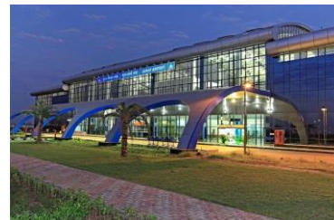
Surat International Airport
