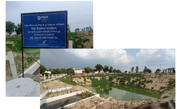
Construction of Pond in Meerut (Rajpura Village)
