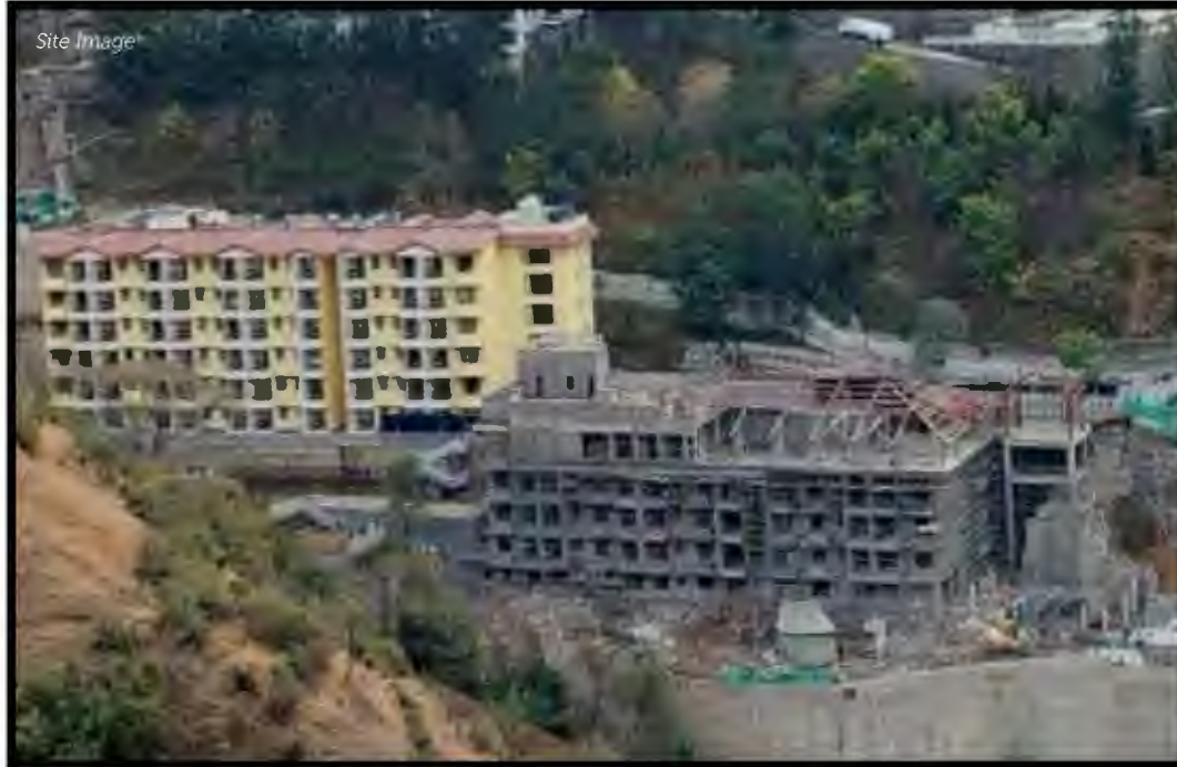
Kandaghat, HP (102 keys expansion) Ph1 (80 keys) completed, Ph2 completion in FY26
