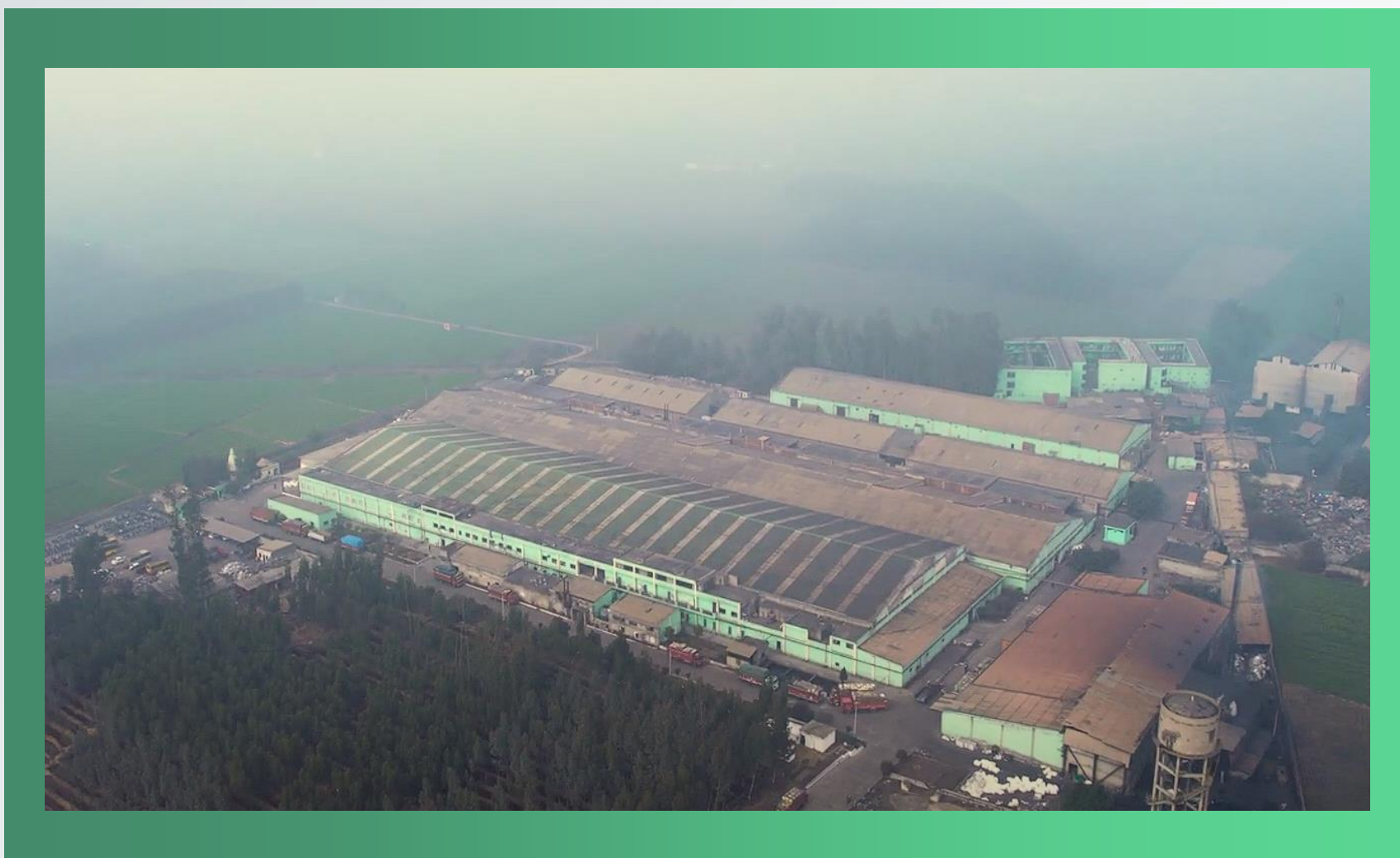
Drone Picture of Shiva Textfab Ltd. based in Ludhiana, Punjab, 100-acre state-of-the-art facility proudly stands as India's preeminent integrated manufacturing unit for rPET waste recycling
