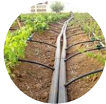
Drip Irrigation Pipes
