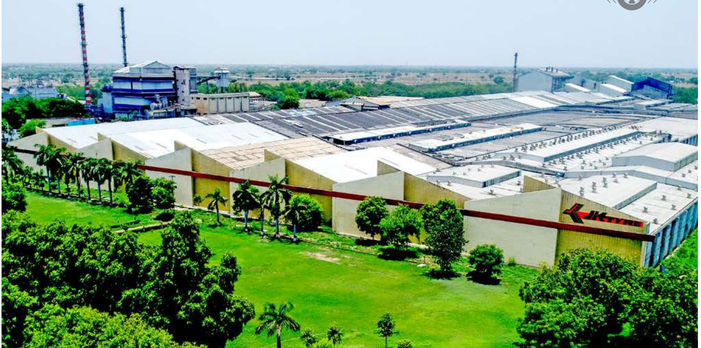
Banmore Tyre Plant
