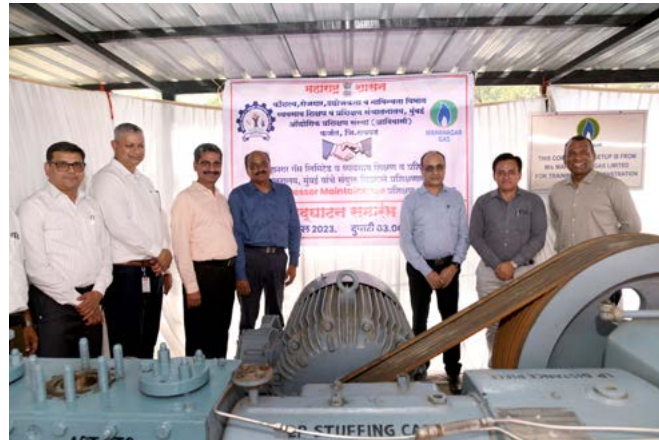
Installation of gas compressor at ITI Karjat.
