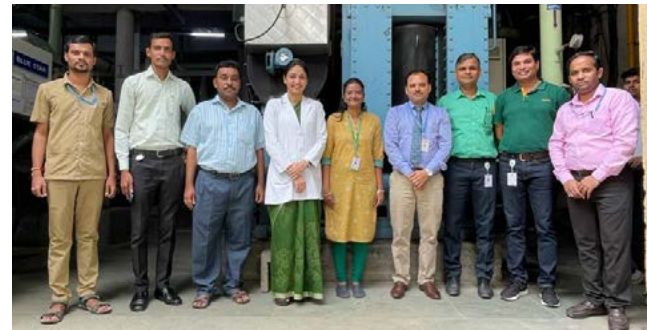
Inauguration of VAM machine at Bai Jerbai Wadia Hospital
