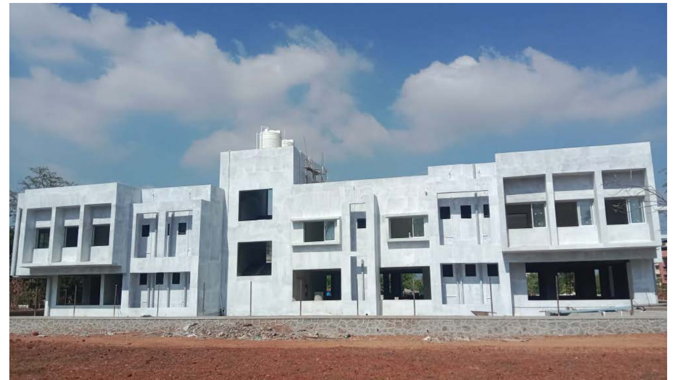
Training centre under construction at Mangaon, Raigad
