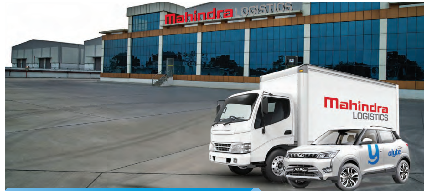
MAHINDRA LOGISTICS STATE-OF-THE-ART BUILT TO SUIT FACILITY AT TAURU ROAD, HARYANA
