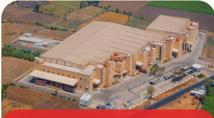
Wagh Bakri Plant
