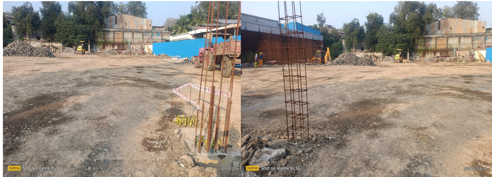
Extension of existing plant to cater to EV OEM
