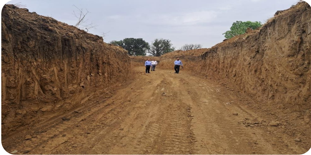
De-silting of 145-meter waterways channel at Bamhauri
