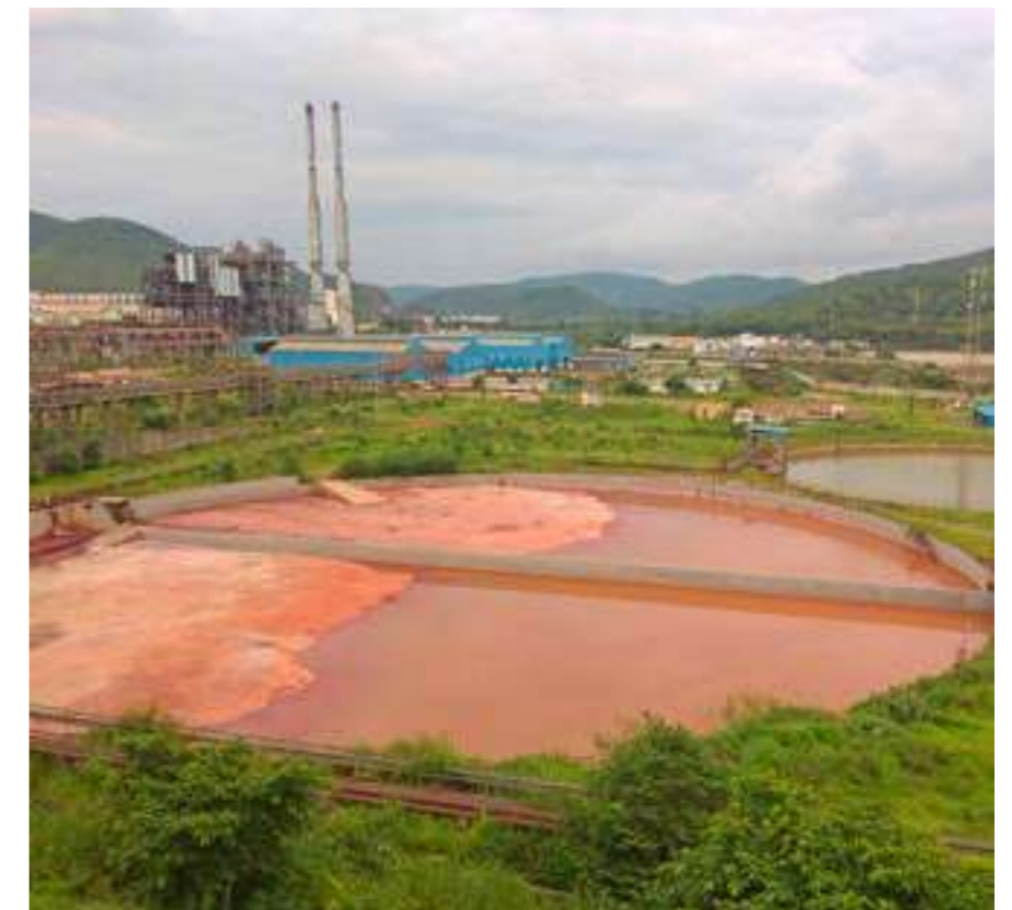
A caustic pond at Utkal Alumina. This pond re-circulates used caustic liquor from the Bayer process
