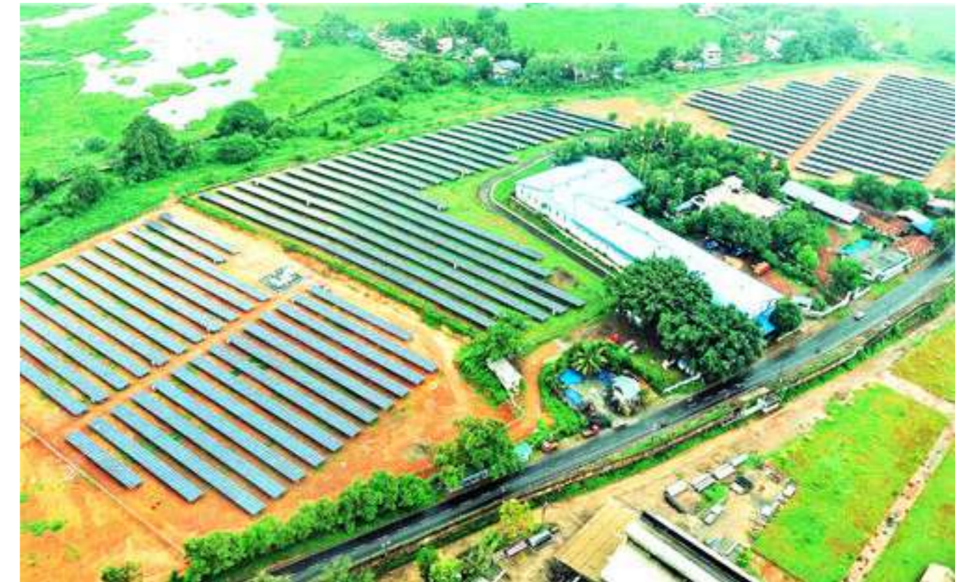
Solar Plant at Alupuram
