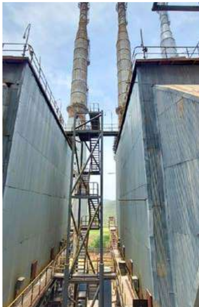
Calciner stack and ESP at Utkal Alumina
