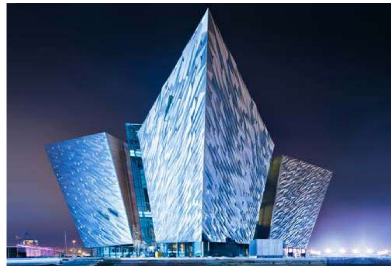
The Titanic Signature Building in Belfast, Ireland, is clad in more than 120 tons of Novelis J57S® anodized Aluminium
