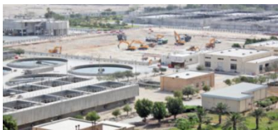
Water Treatment Plant, Doha
