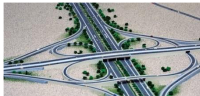
Sheikh Khalifa Interchange, UAE
