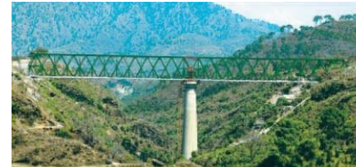
88m Rail Bridge Jammu Udhampur
