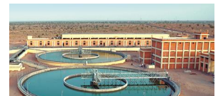
Water Treatment Plant, Barmer
