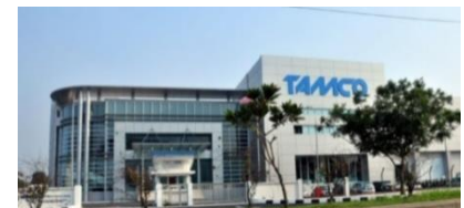
MV Switchgear Factory, Malaysia
