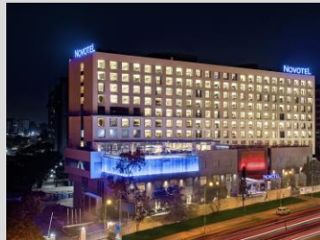
Novotel Pune Nagar Road 311 Keys
