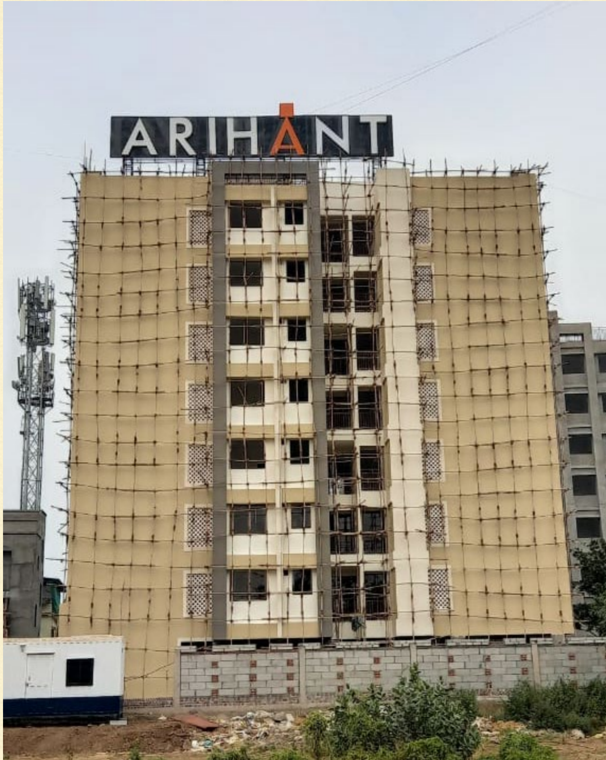
Flooring & Tiling, Doors & Windows completed
