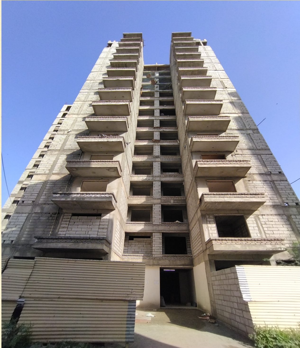
15 th Slab work in progress
