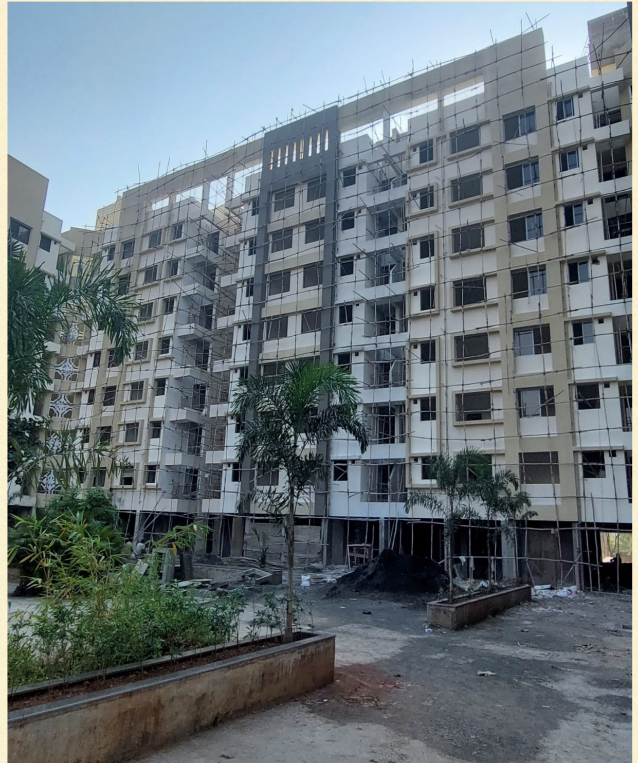
Flooring & Tiling completed
