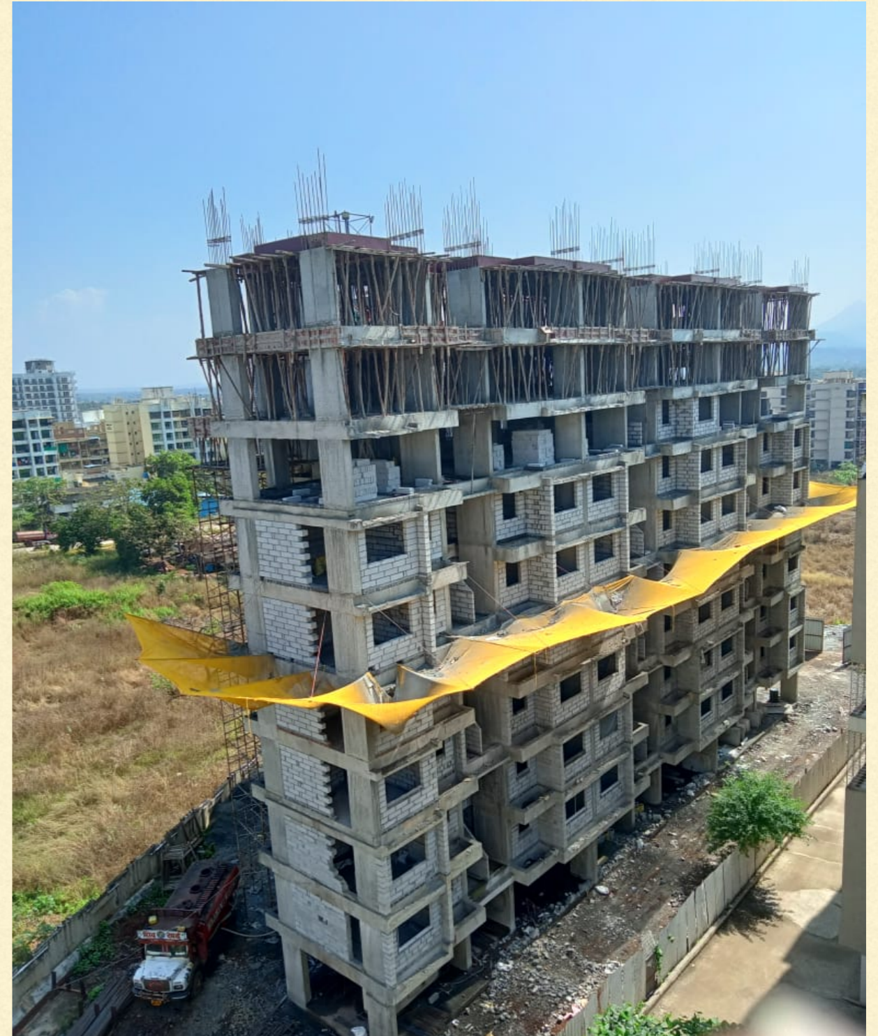
RCC work up to 9 th slab level completed
