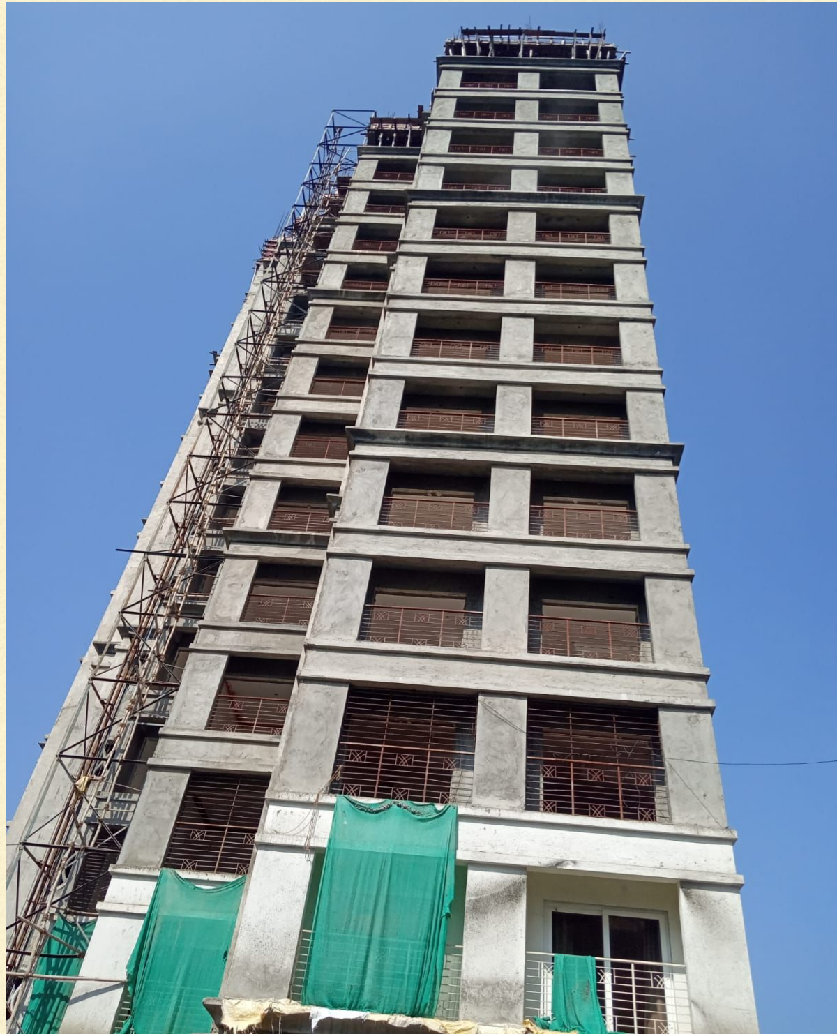
Flooring, tiling, kitchen works in progress
